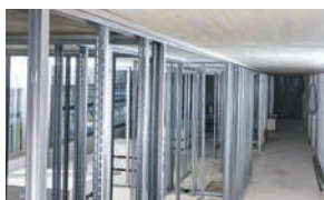
Drywall tracks to concrete and steel
