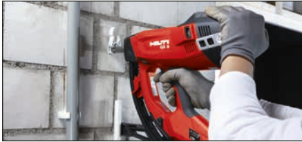
Conduits and light-duty pipes
