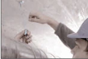
Round Air Ducts
