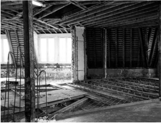
Figure 103. Application of shear connection for building renovation
