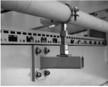
Figure 87. Fastening of brackets with blunt-tip threaded studs
