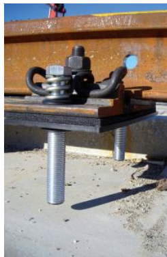
Clipped components before concrete pouring
