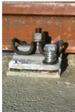
Support after concrete pouring
