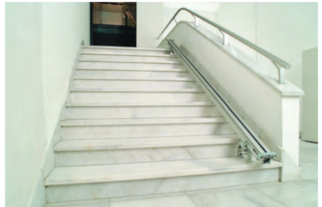
Installation of rail supports for angular cutting and cutting on stairs
