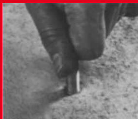
Screw the threaded rod in internally threaded anchors such as the HKD (HDI) or TDD (HSS). In the case of the HSL replace the bolt by the threaded rod.
